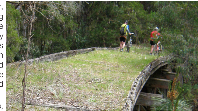
Bridges over deep gullies were helpful
